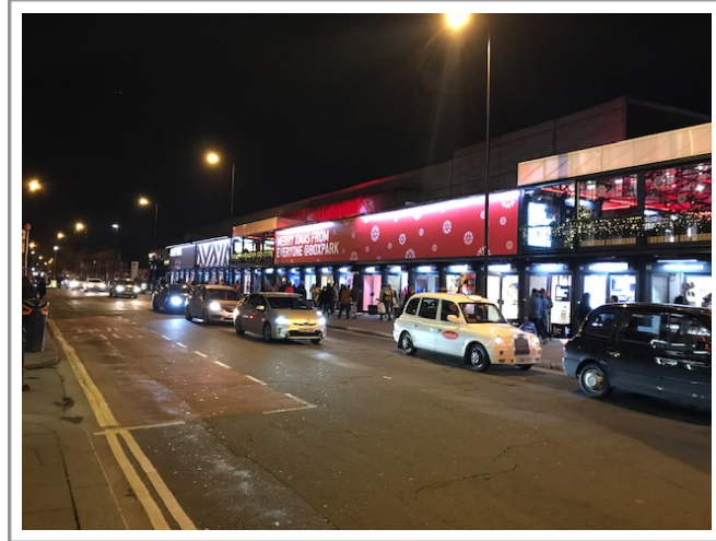
Shipping containers were used in this project in London to create a fast and inexpensive development. Shipping containers have been used for permanent and short-term projects. These could be used on the South side of Union Avenue area under the Route 34 overpass (opposite the SITE Project installation) to create stores and restaurants to activate the street and make it safer. Photo by Christopher Bergstrom.
